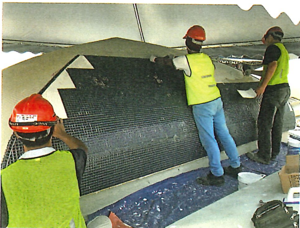
The installation of new glazed porcelain mosaics on the dome was carried out from the bottom layer and working upwards.
