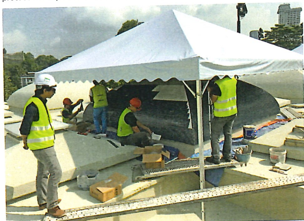
Temporary tents were erected to cover each dome and pyramid roof during the mosaic installation stage in order to protect them from direct sunlight and heavy rain.
