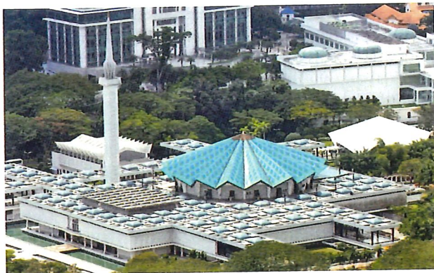
Built in 1965, the National Mosque (or Masjid Negara ) features a 73 m-high minaret and an 18-pointed star concrete main roof reflecting an open umbrella, while the cap of the minaret resembles a folded one.
