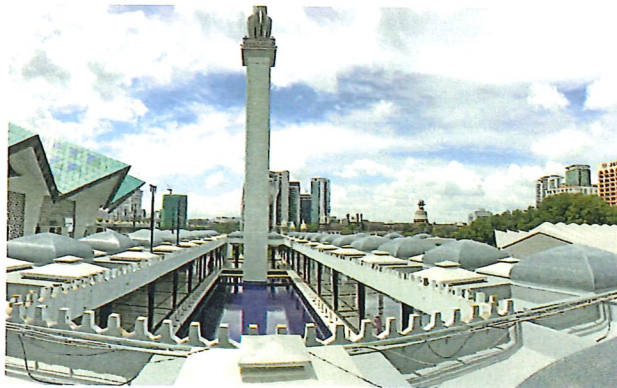
Upon completion, a total of 13,482,953 new glazed porcelain mosaic pieces were used to cover 95 domes and 270 pyramid roofs on the flat roofs of the National Mosque.
