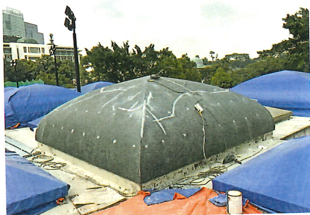
The dome after completion of work using the "Helifix-DryFix" stainless steel helical pinning system.
